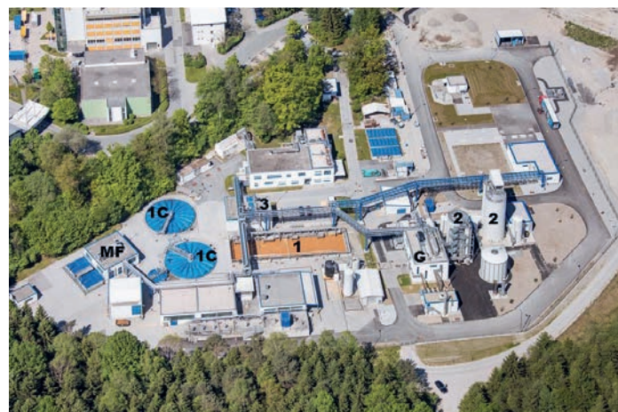
Fig. 3. Aerial view of the Roche Penzberg WWTP. (1) Serial open air-fed aerobic biodegradation tanks, (1C) covered air-fed aerobic biodegradation tanks. (2) Anaerobic digester towers. (3) Closed, pure-oxygen-fed biodegradation. G = Biogas electricity/steam co-generation. MF = Membrane filtration for activated sludge. Photo ©Roche Penzberg.
