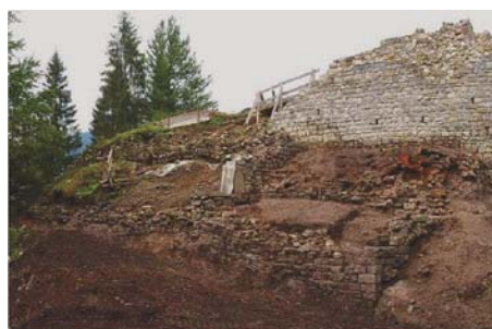
Fig. 4. The Medieval Sachuidic castle, Friuli, Italy, before restoration. The cluster analysis of the XRPD spectra of the mortars (Fig. 6) allows the detailed interpretation of the different building stages throughout the history of the site (Fig. 7).
