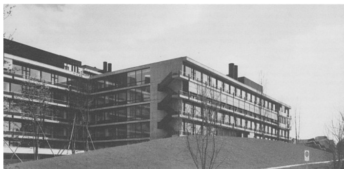
Fig. 22. Winterthurerstrasse 190; part of buildings 32 (left) and 11 (right)
