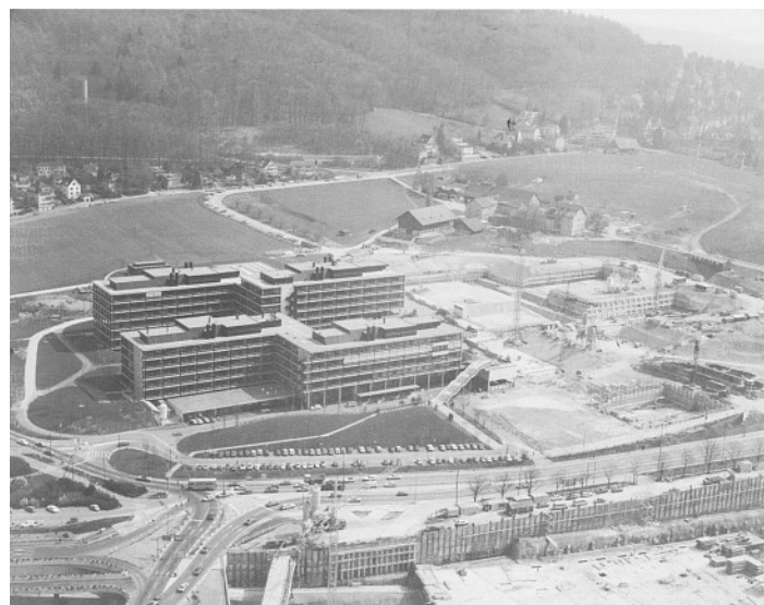
Fig. 23. Overhead view of the University of Zurich Irchel, first stage (photo by Swissair)
