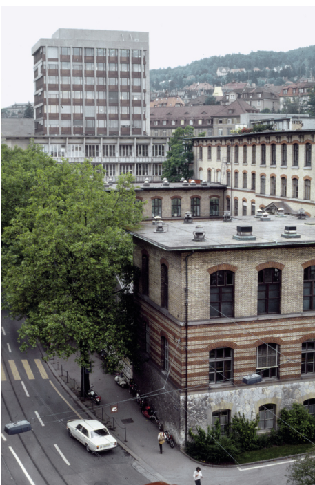
Photo 2. Chemistry Buildings on Universitätsstrasse
