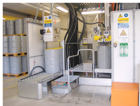
Fig. 4. Fully automated multi-product drum filling station
