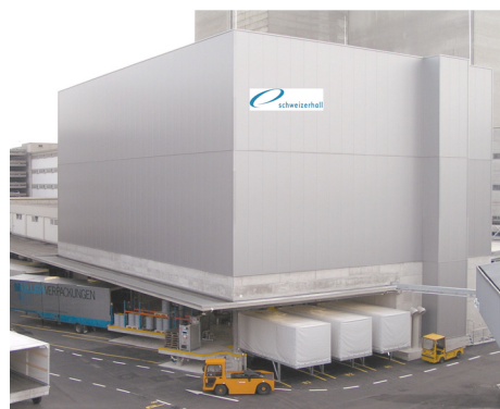
Fig. 3. Compact high-bay warehouse for flammable solvents
