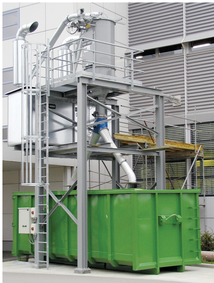
Fig. 3. Glass tip removal set-up outside the production building
