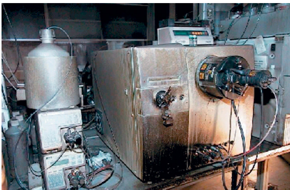
Fig. 2. Property damage by smoke impact on expensive LC-MS equipment
