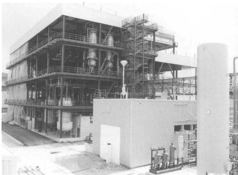
Fig. 6. View of the production building (imine preparation, hydrogenation, distillation). The small building in the foreground houses the hydrogen compressors.
