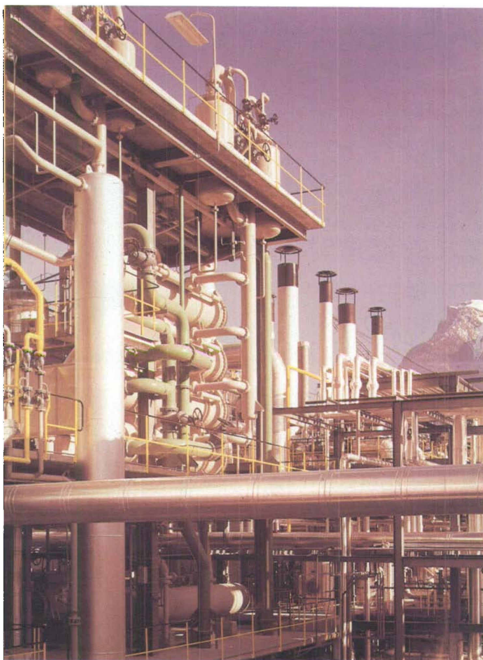
Fig. 2. In the late 1950s, Lonza decided to use oil rather than calcium carbide as its raw material. In the fall of 1964, Lonza brought on stream the world's smallest industrial naphtha cracker in Lalden.
