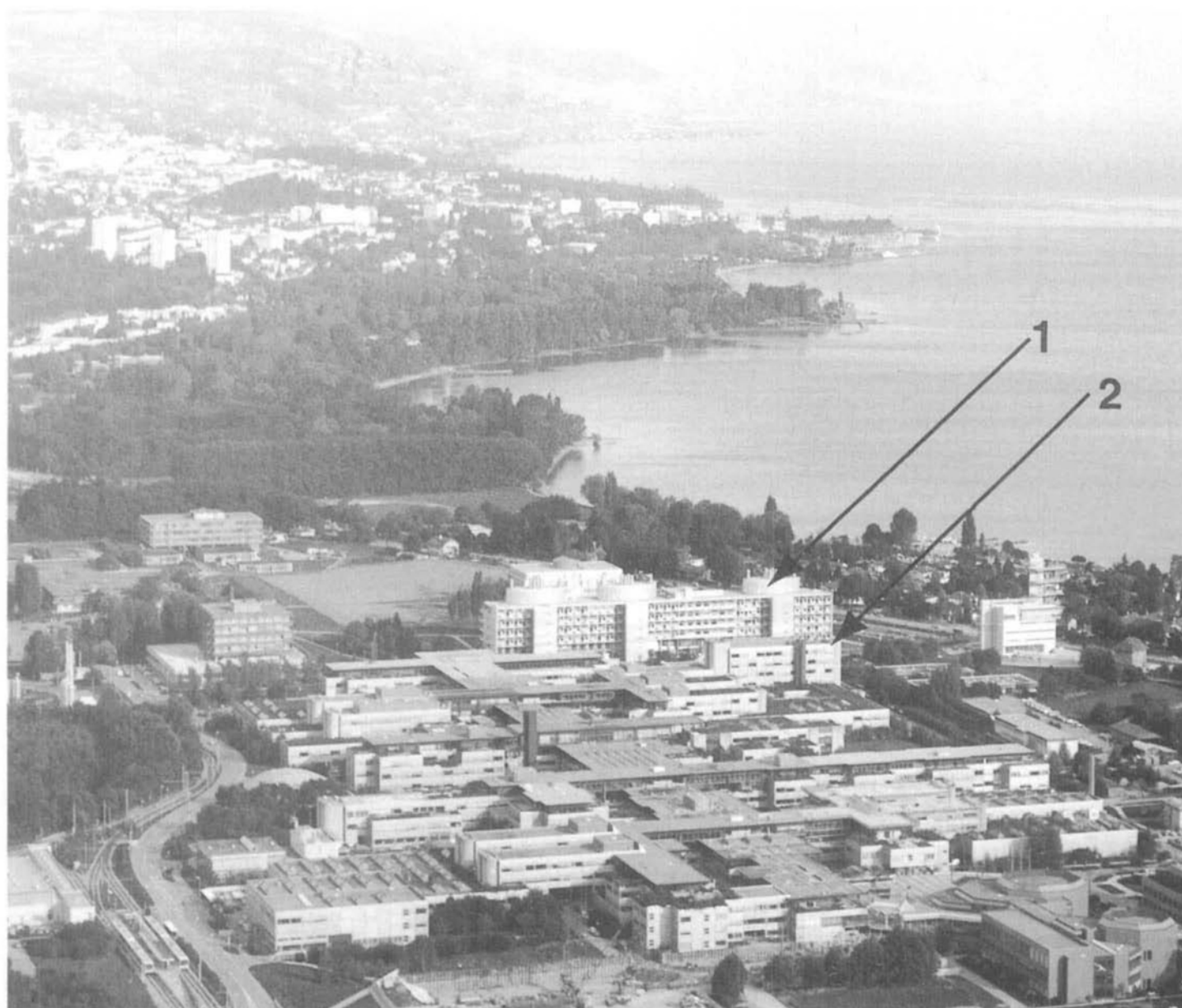
Fig. 2. Forming a single site, 1) the new Chemistry building of the University and 2) the chemistry area of the Swiss Federal Institute of Technology (photo: A. Herzog)
